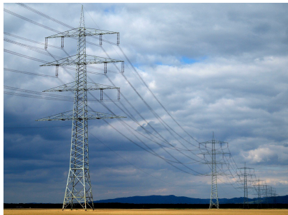
Triple-circuit 400 kV overhead line with 4 conductors per phase
